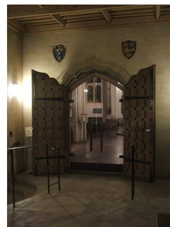
Glazed doors in existing door reveal combining transparency and security ( St Edmundsbury cathedral)
