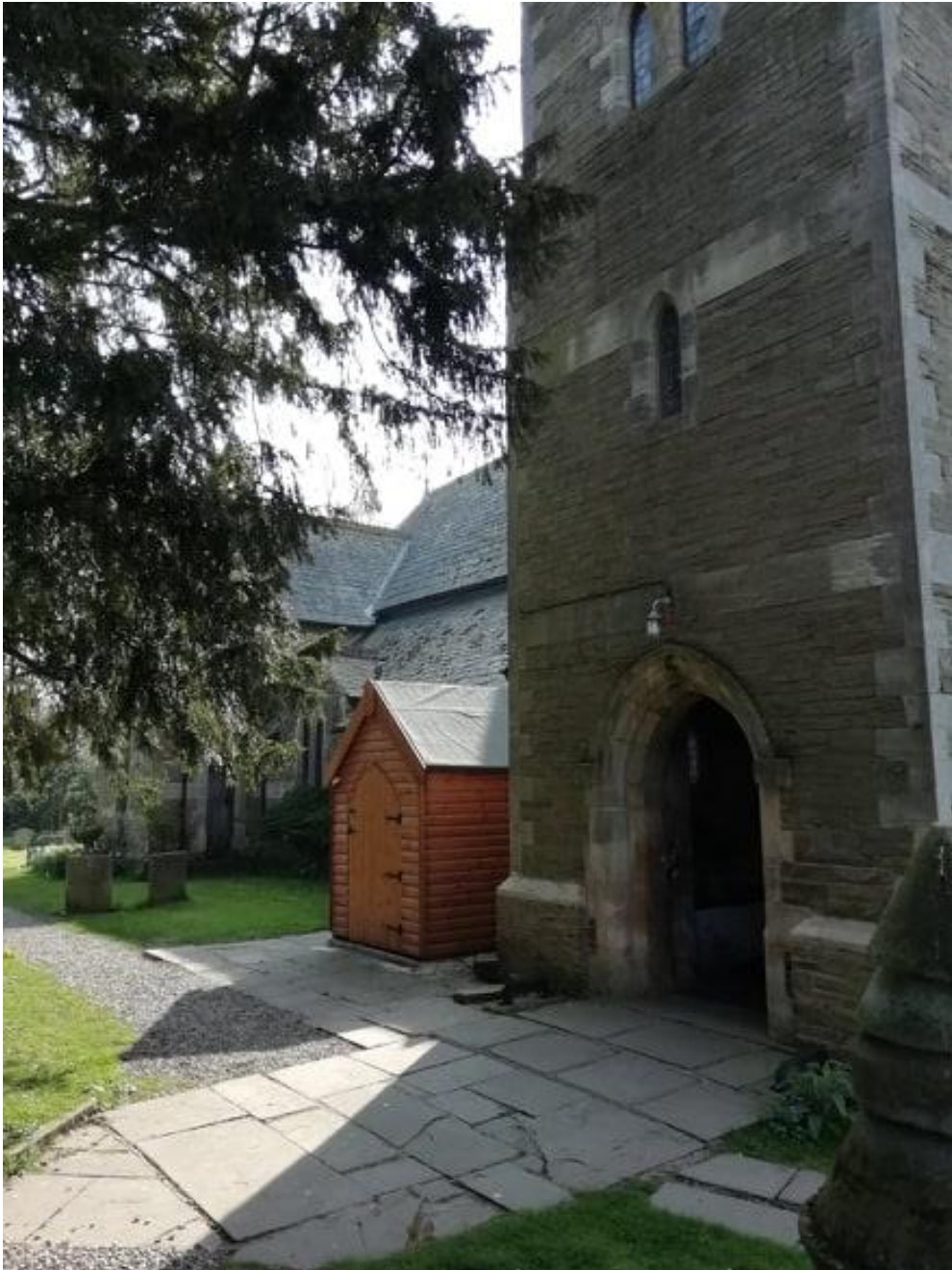
Self-composting WC within the church yard of Elvington Holy Trinity
