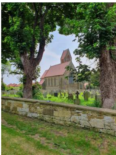
a) North boundary in fair condition
