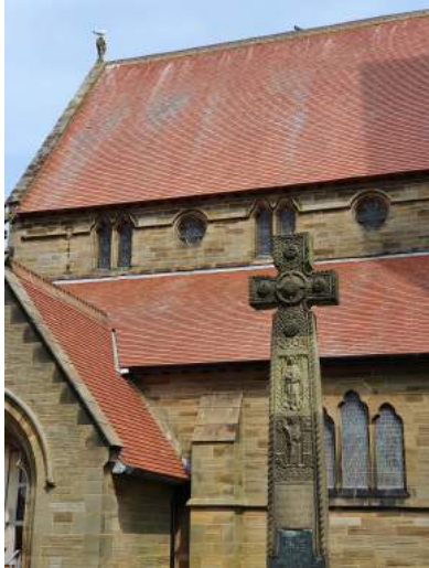
a) Tiles to repair on the Nave south slope
