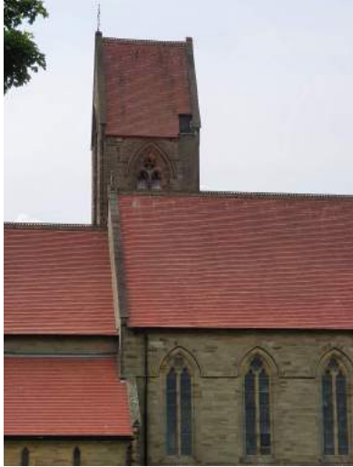
a) Access door is visible at the eaves of the north slope of the tower roof
