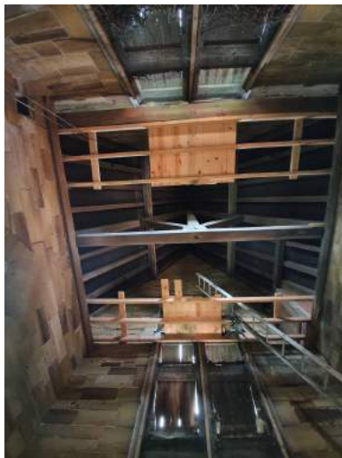
a) Roof structure
