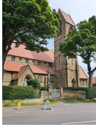
b) The height of the tower creates restricted view of the south roof slope of the tower
