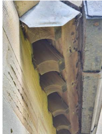
b) Exposed rafter ends in fair condition.
