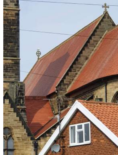
b) South slope viewed from the SE.
