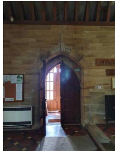
b) South entrance door
