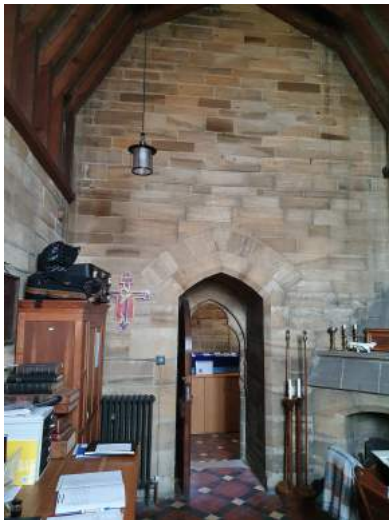
a) Entrance from tower base. Historic staining/ funnel marks at high level. Fireplace in right of photo.
