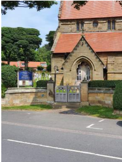
a) South gates – main entrance
