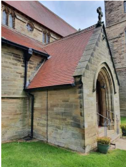
a) SW view of porch
