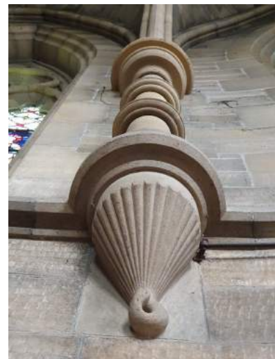
b) Fine carving to pilaster corbels
