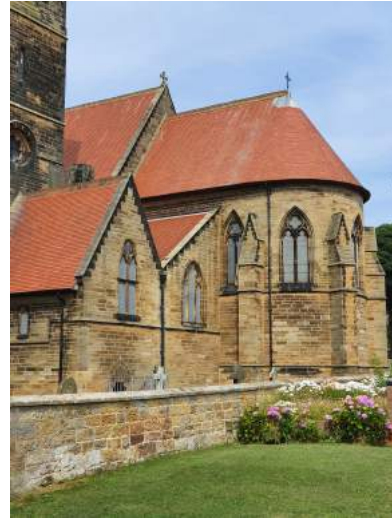
b) The Chapel and Vestry roofs form a valley gutter and are adjoined to the chancel/ Sanctuary
