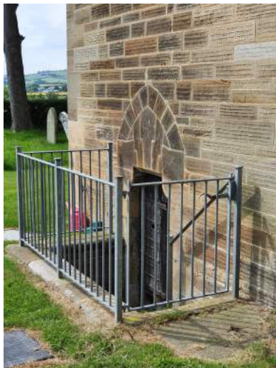
a) Basement Access
