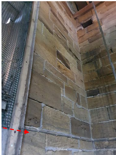
a) Note the light grey cement based mortar
