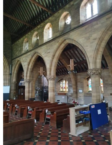
b) South aisle viewed from the Nave
