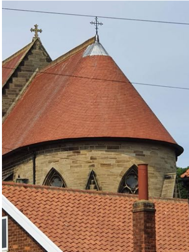
a) Apsidal roof at the east end over the sanctuary
