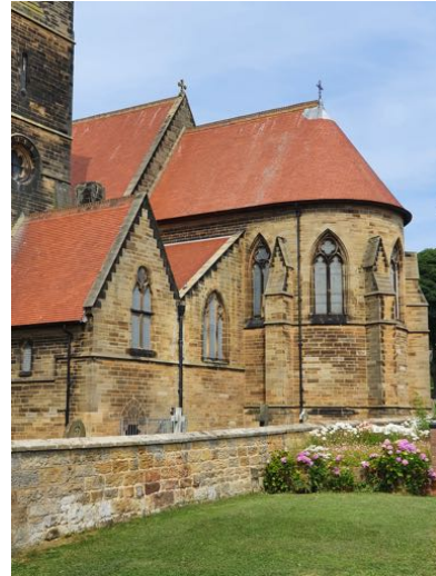
b) The Chapel and Vestry roofs form a valley gutter and are adjoined to the chancel/ Sanctuary
