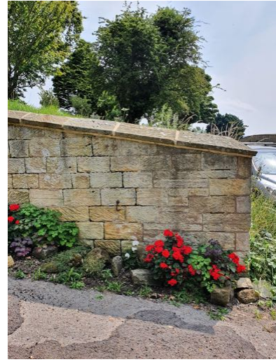
b) Coping stones recently re-bedded.
