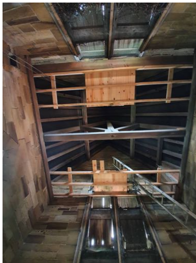
a) Roof structure
