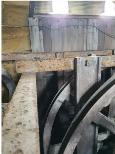
a) Bell frame corrosion
