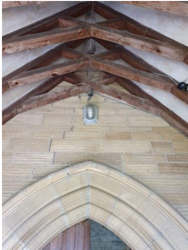
a) Porch doors
