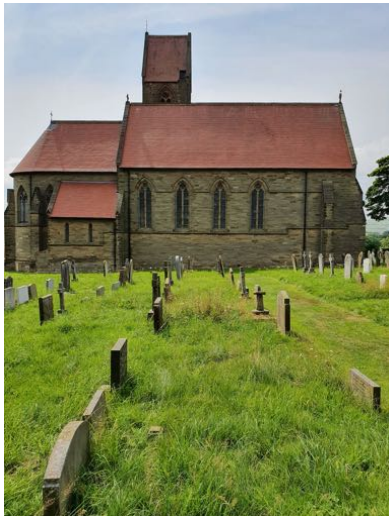
a) View from the north
