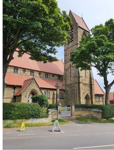
b) The height of the tower creates restricted view of the south roof slope of the tower
