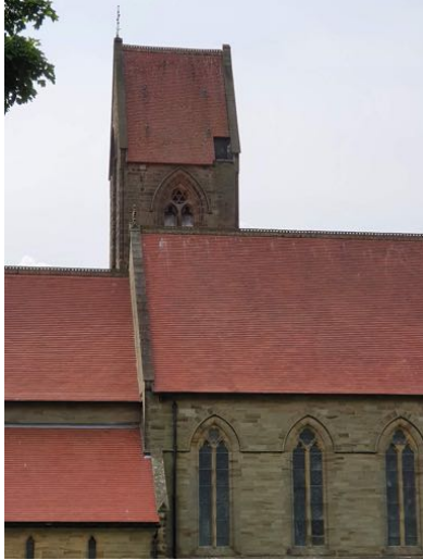
a) Access door is visible at the eaves of the north slope of the tower roof
