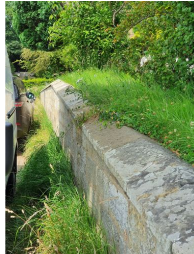
b) South boundary wall retains the raised churchyard
