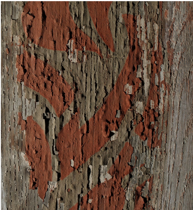
Damage to a painted ceiling and salt deterioration on masonry due to unstable environmental conditions.
