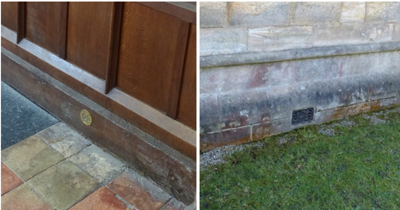
External and internal ventilation openings to under pew voids are designed to reduce moisture levels.
