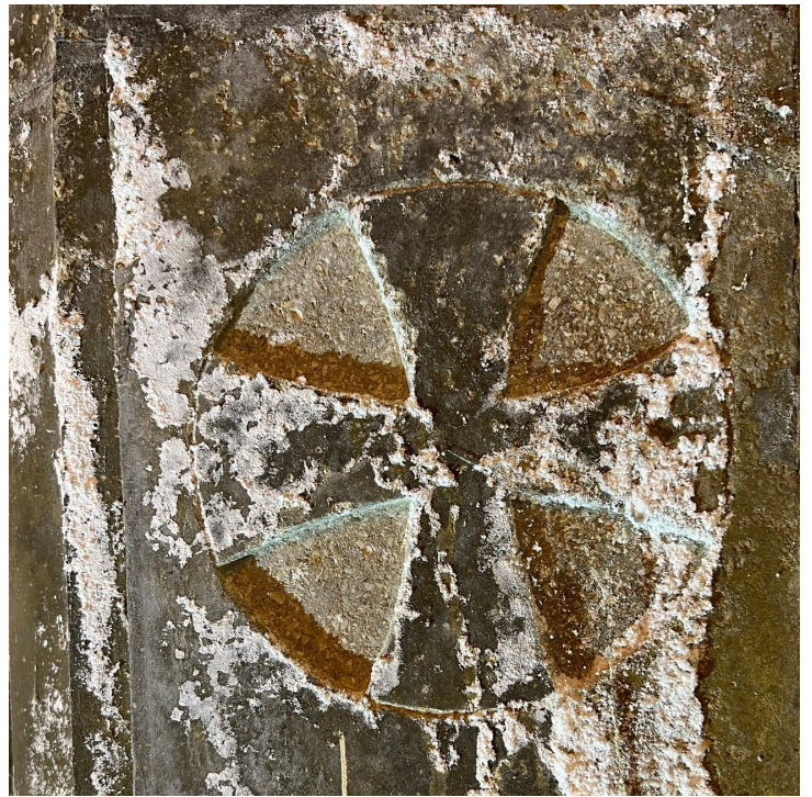
Damage to a painted ceiling and salt deterioration on masonry due to unstable environmental conditions.
