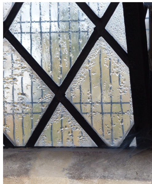
Severe condensation can form on cold surfaces, such as glass, causing damage to adjacent stonework.
